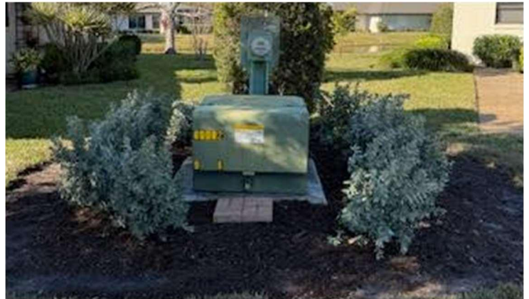
Figure 5 - FPL Vault After (Mock-Up in Progress)
