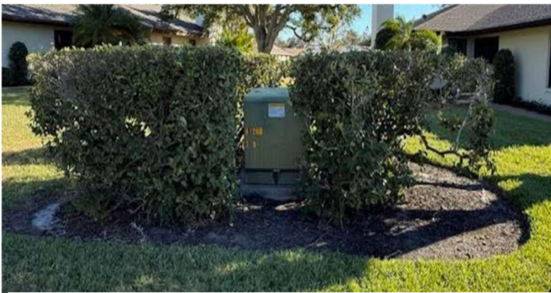
Figure 6 - FPL Vault (Before)
